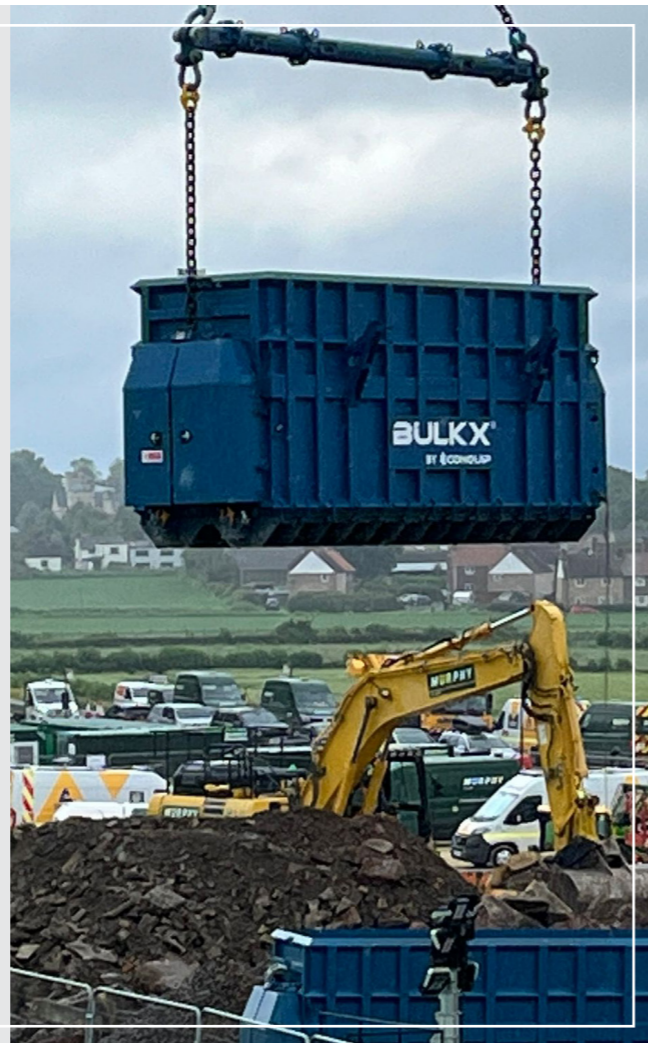
TRANSPENNINE ROUTE UPGRADE | TRU EAST ALLIANCE
