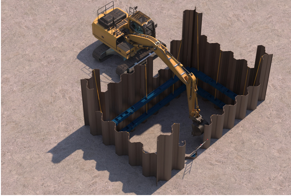
07. Upon reaching the level for the next frame. Assemble legs and lower onto timber skids, positioning tight to the sheets and ensuring tolerance to swing in the last corner. Check frame is level and pack it as required. Once all legs are in position, pump out each corner ram to approximately 100 Bar and attach restraining chains.
