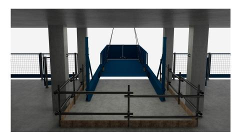
20. Manoeuvre the deck as far back into the building as possible and lower onto the slab so that both beams are flat.
