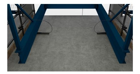
29. Continue to lift the deck until you have a gap high enough to position 2 short scaffold tubes under each beam, securing with a tether.
