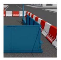
15. Prior to lifting, ensure tag lines are attached on the front and near the top of the deck on the rear, so they can be removed once installed.
