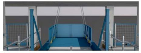
7. Re-insert the prop pins and clips, then remove the prop heads.
