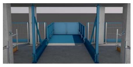
2. Prior to lifting, attach a tag line to the front and rear of the deck in opposite corners.
