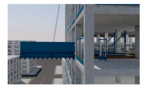
20. Once the platform is butted up against the slab edge, lower off the crane until the beams are sat flush on the slab.
