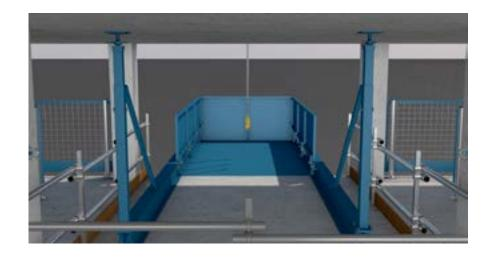
24. Check the screw jacks are tightly secured, slowly lower the crane down and disconnect the lifting chain.
