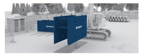
2. Using an excavator or other suitable lifting apparatus, lower the Drag Box into the trench, with a suitably rated 4 leg chain.
