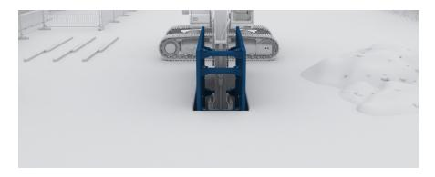
8. Continue to dig in between the panel faces until the desired depth is reached.
