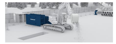
1. Excavate the initial section of the trench to the dimensions (length x width) of the Drag Box base unit Do not dig deeper than the legal limit of 1.2m.
