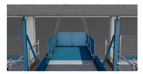
23. Ensure that the base beams are flat on the ground and they vertical legs are at 90 degrees to the base beam. Tighten the screw jacks until they are hand tight, then hammer just 1/4 turn extra.
