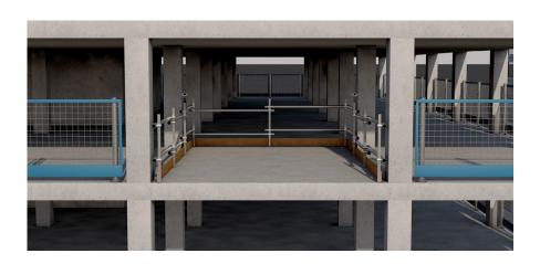
3. Install location will need a suitable anchor point for leading edge safety equipment to attach.
