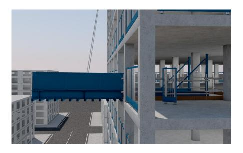
20. Once the platform is butted up against the slab edge, lower off the crane until the beams are sat flush on the slab.
