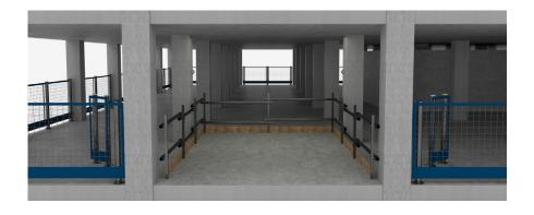
3. Install location will need a suitable anchor point for leading edge safety equipment to attach.
