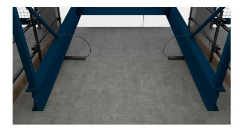
29. Continue to lift the deck until you have a gap high enough to position 2 short scaffold tubes under each beam, securing with a tether.
